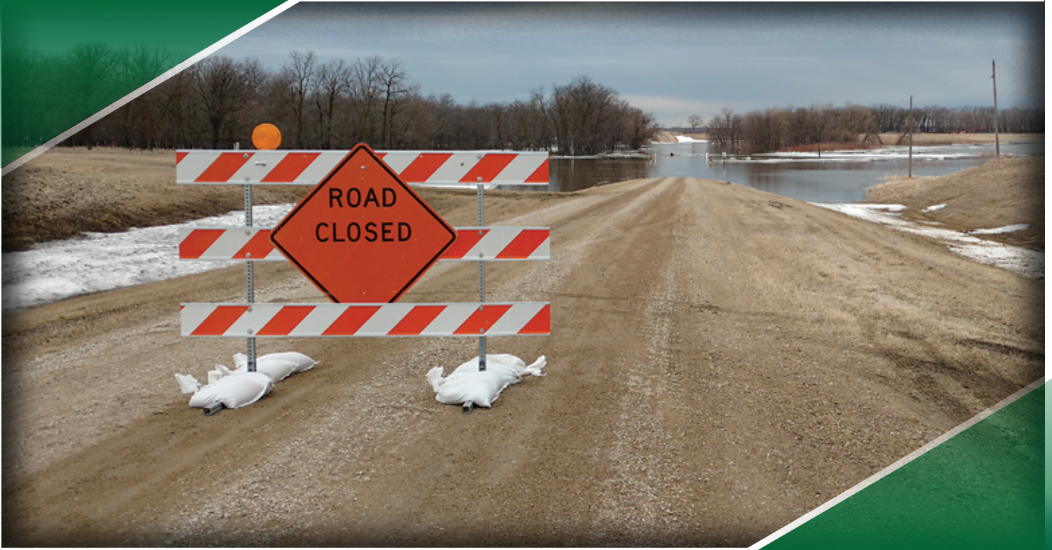
Kittson County flooding closed roads in March 2017.
