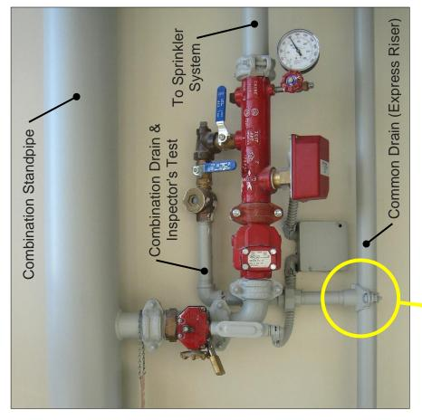
**NOTE:** Common drain riser properly sized larger than system drain.
