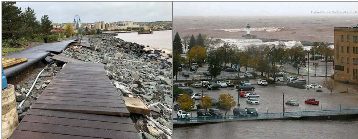
Figure 60. Wave Action and Flooding in Duluth's Canal Park, October 2018.
