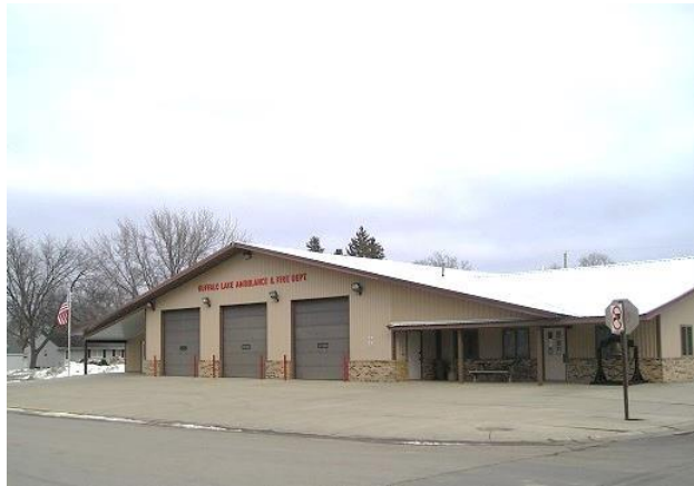
Figure 16: Buffalo Lake Fire Station
