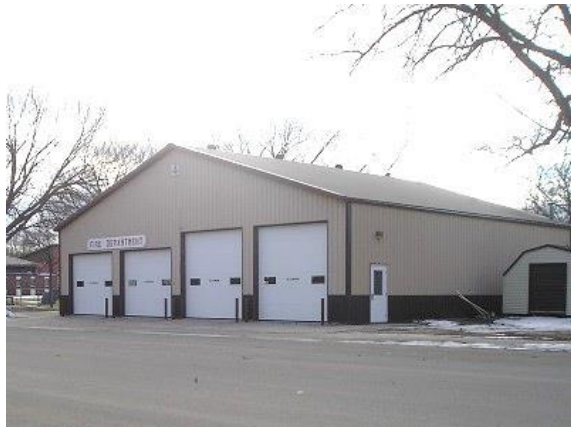
Figure 18: Franklin Fire Station
