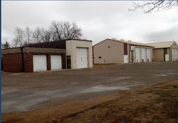
Figure 25: Milaca Fire Station
