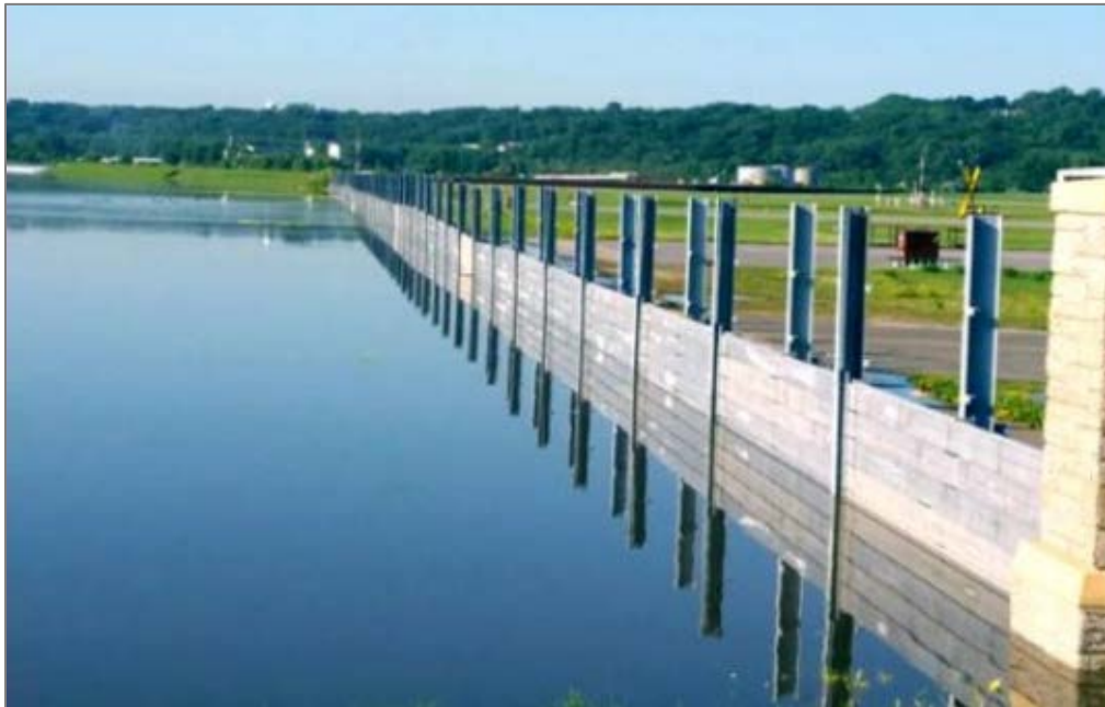
Figure 74. Removable Floodwall at the St. Paul Holman Field
